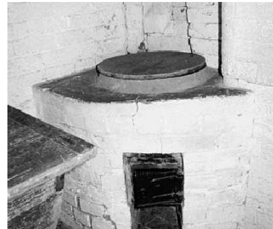
A copper to heat up the water.
